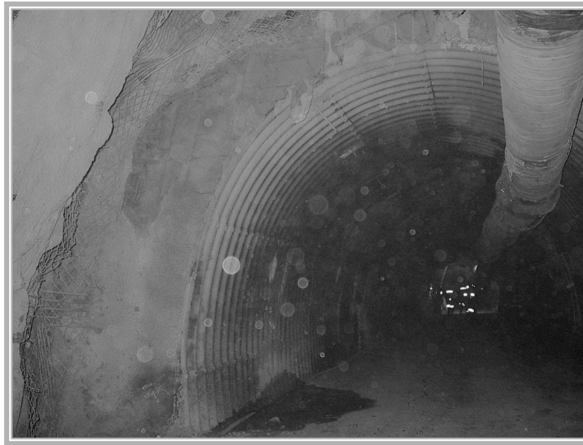
Figure 16. Void Filled with Aerated Cements.
