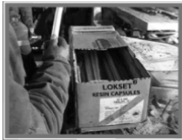
Figure 12. Lokset® resin Capsules.
